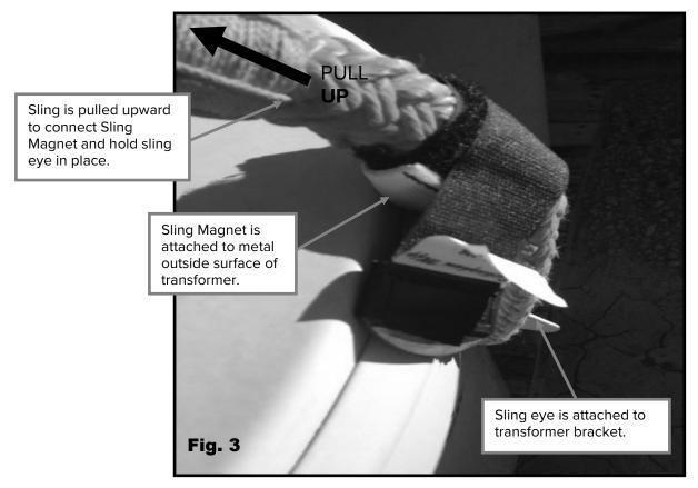
Step # 5 – With the first sling leg secured by the Sling Magnet, attach the other sling eye to the opposite transformer bracket. You have now completed the sling attachment procedure utilizing the Sling Magnet (see Fig. 4):
